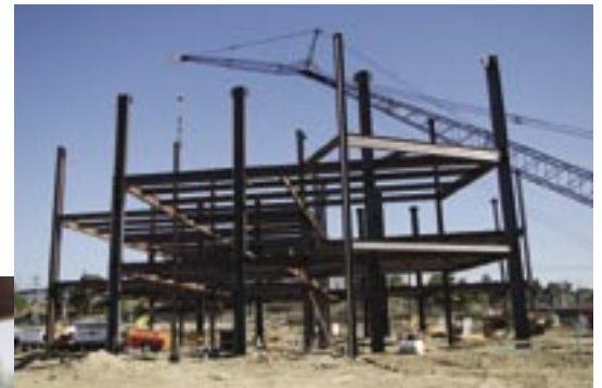
Workers finish installing the structural steel and flooring deck on The Joe & Vi Jacobs Community Center.
