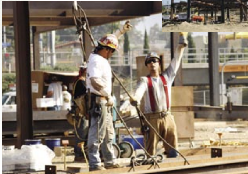
Workers finish installing the structural steel and flooring deck on The Joe & Vi Jacobs Community Center.
